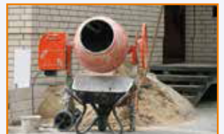
Cement & concrete production
